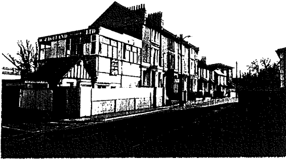
92-95 Parrock Street are of interest but contrast with much of Windmill Hill
