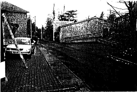
Kingdom Hall's side elevation would be enhanced if the car park were landscaped
