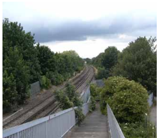
Figure 16. Pedestrian bridge over the railway at Mark Lane
