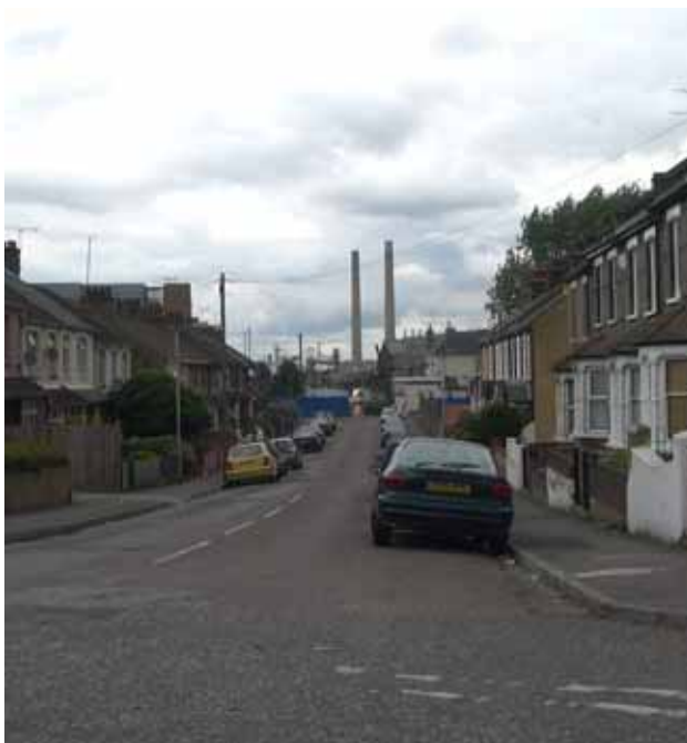
Figure 28. View of the power station along Russell Road
