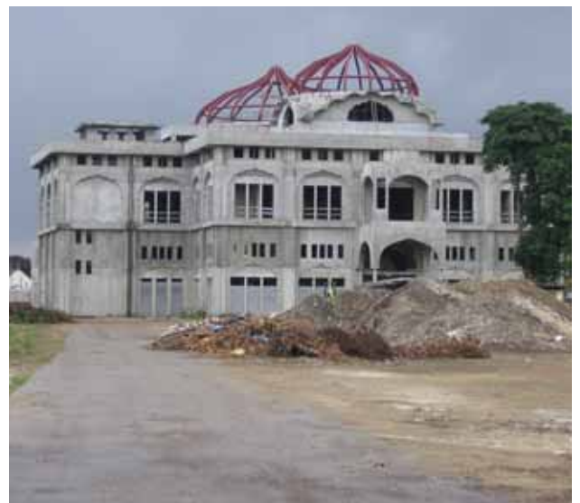
Figure 18. The Siri Guru Nanak Darbar Gurdwara under construction
