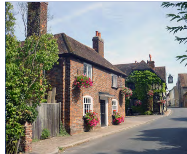
Traditional metal frame leaded light casement windows above timber sliding sashes - Cobham Conservation Area
