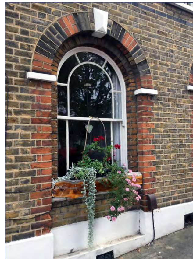
Original timber arched sash window - Windmill Hill Conservation Area
