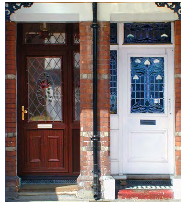
Example of a modern double glazed uvpc door next to a timber door with original stained and coloured glass in an urban Edwardian terrace.
