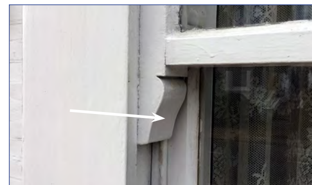
Horn - common feature on sash windows from the Victorian period onwards.
