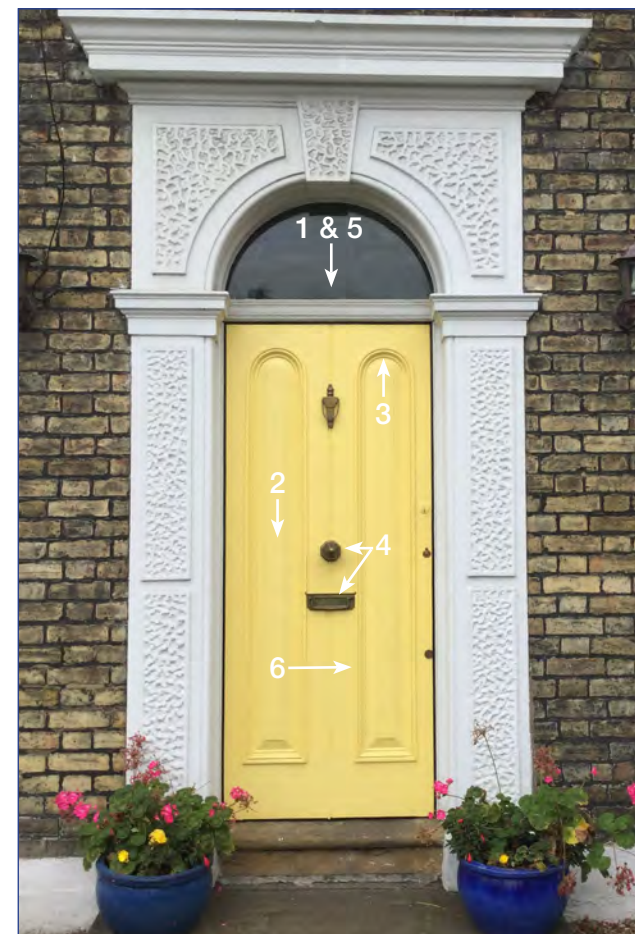
1. Fanlights, 2. panelling, 3. Moulding style and depth, 4. Door furniture; letter box, door knocker etc, 5. Glazing, 6. Traditional painted finish (not stained or varnished)
