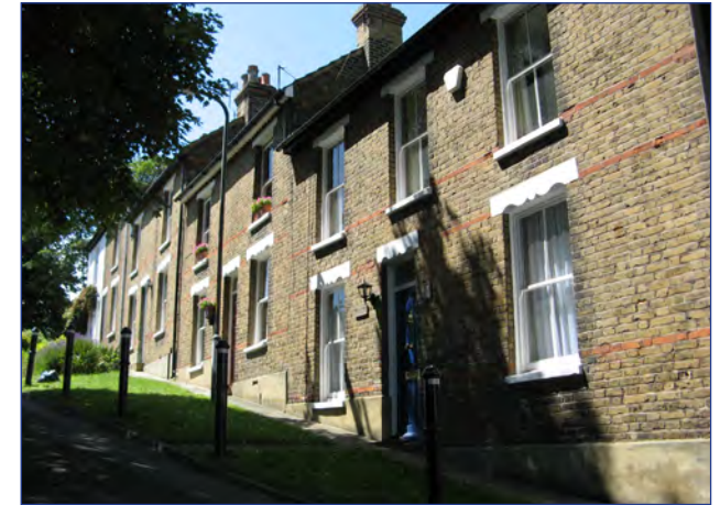
Timber sash windows
