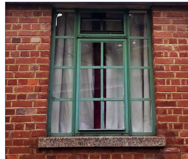
Historic metal casement windows still survive in urban and rural Conservation Areas - High Street Conservation Area
