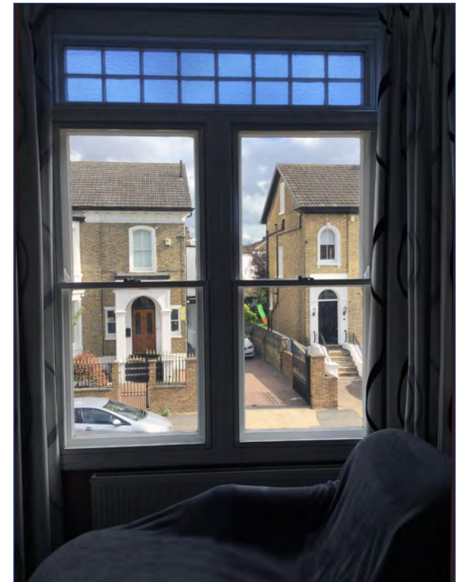
Example of well fitted secondary double glazing with proportions matching original window dimensions and glazing details - Darnley Road Conservation Area
