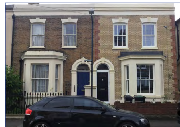
Use of approved replacement windows in non traditional material reflecting the proportions and style of the adjacent property - Darnley Road Conservation Area.
