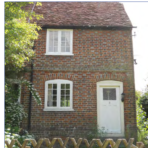
Timber casement windows
