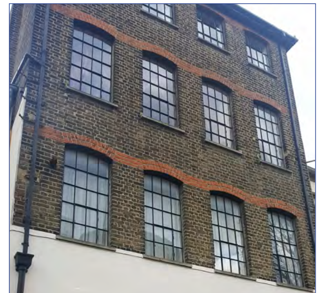
Cast iron windows - High Street Conservation Area
