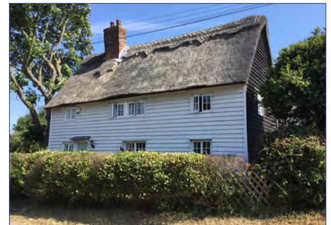
Original timber casements - Church Street, Higham Conservation Area
