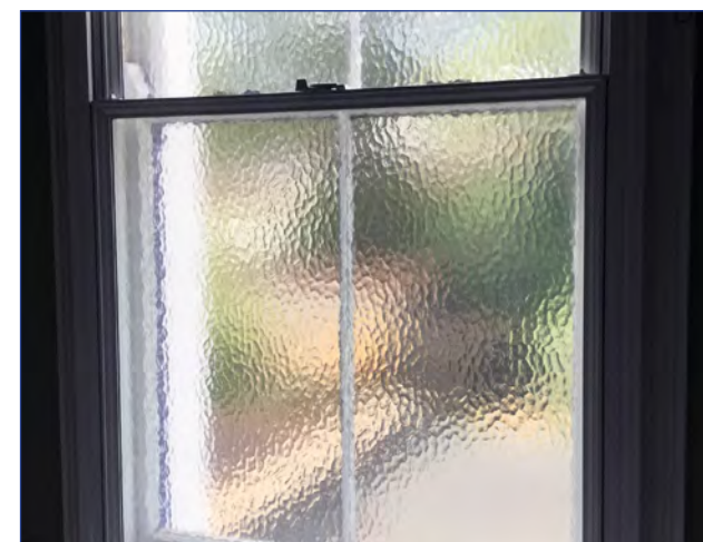
Secondary glazing designed to open by the same method as the external window.
