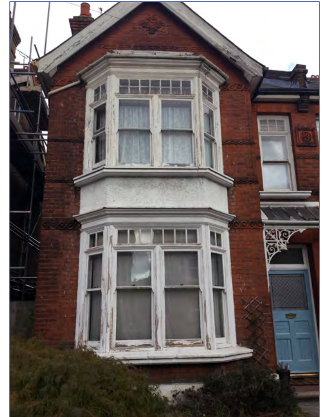
Removing old paint from windows and doors as part of a maintenance routine will allow you to assess for repairs.
