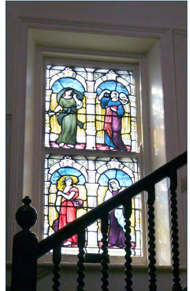
Example of existing original stained and coloured glass. It is important to retain original glazing when replacement is necessary as modern double glazing cannot replicate originals.
