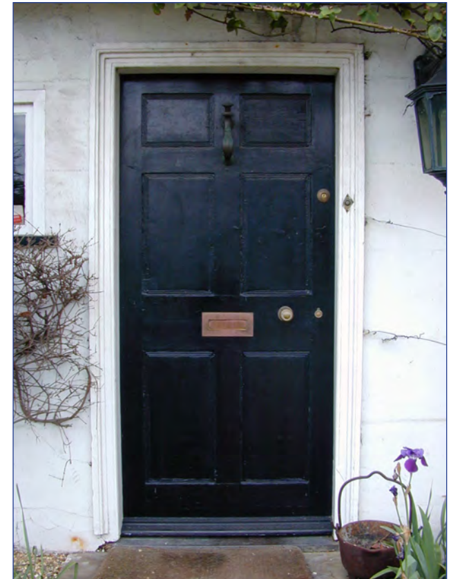
Traditional timber panelled door - Thong Lane Conservation Area
