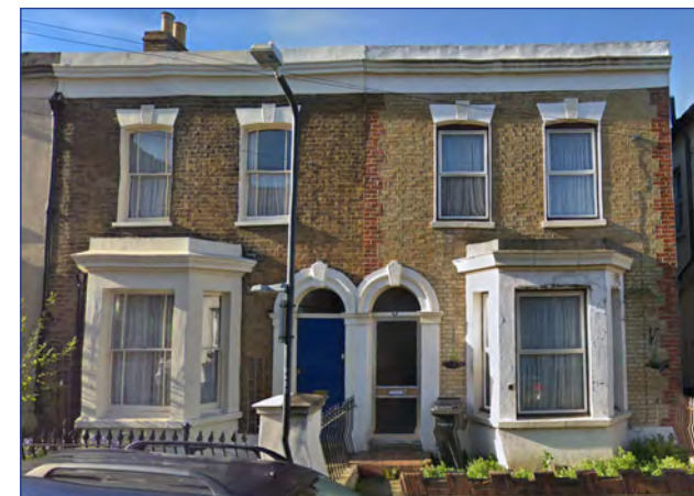
Property before replacement windows and door. (on right)
