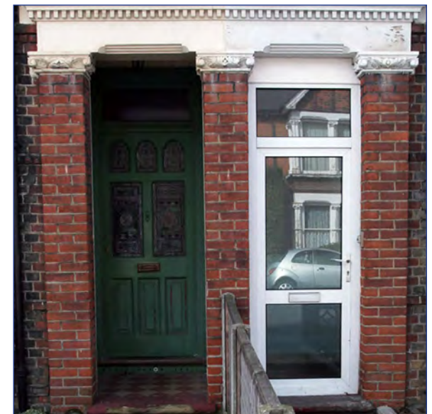
Enclosing recessed doorways detracts from shared features and the area's character.
