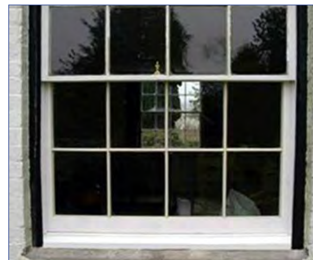
Like-for-like repairs do not require planning permission.
