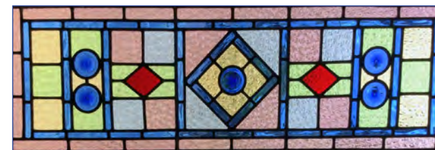
Detail of original stained and coloured glazing in an original timber door in an urban Edwardian terrace.
