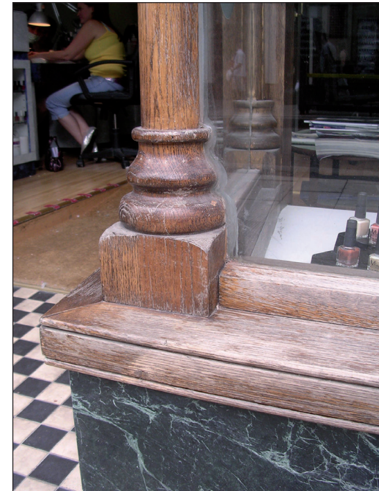
Example of a stained shopfront sill that has prematurely greyed and faded. Additional coats need to be applied to horizontal surfaces or areas of high sun exposure to ensure that they weather evenly with other parts of the joinery.
